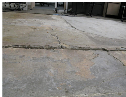
Building E structural movement evidence
